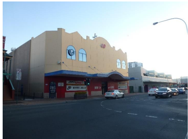
Figure 7: Commercial building occupying the site as viewed from Scott Street (north east)
